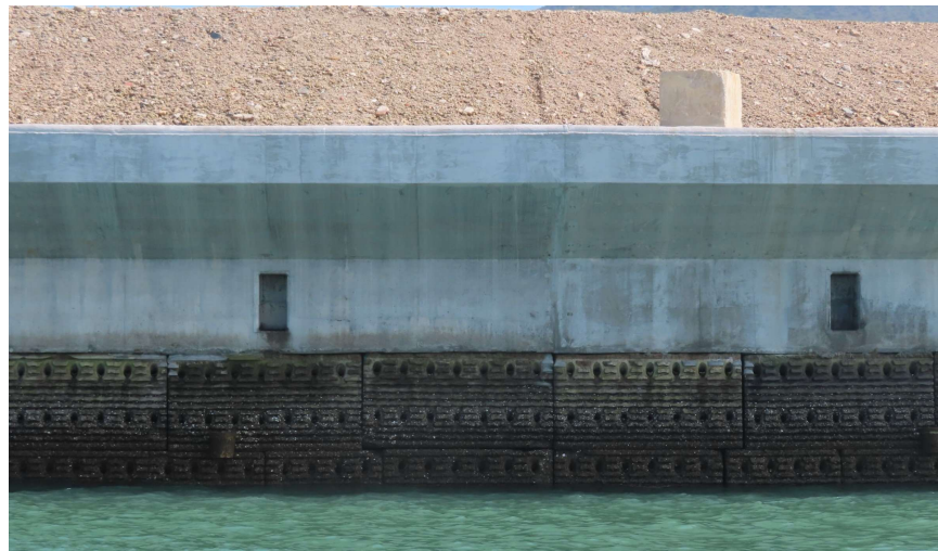
General View of Vertical Eco-shoreline
